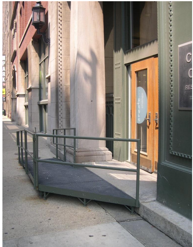
Side portable ramp has been installed to make this college entrance accessible
